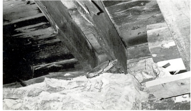
First floor joists, sill-plates and rough flooring were badly rotted or warped and required costly replacements.
