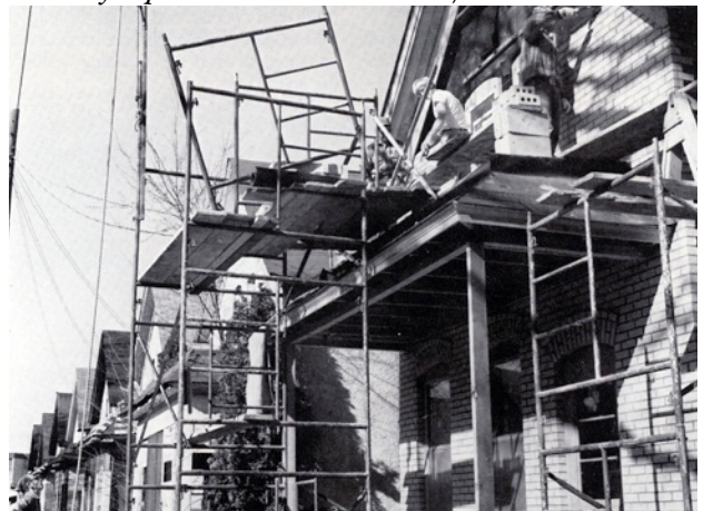
Both new and used brick has been used to match the originals as closely as possible. This scene is at 2017 Milwaukee
