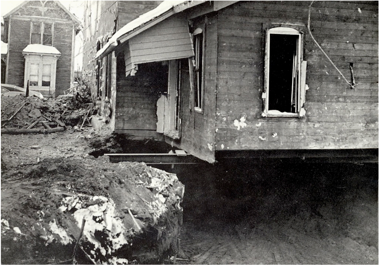
Deterioration of the original stone foundation required replacement with contemporary cement block basements.
